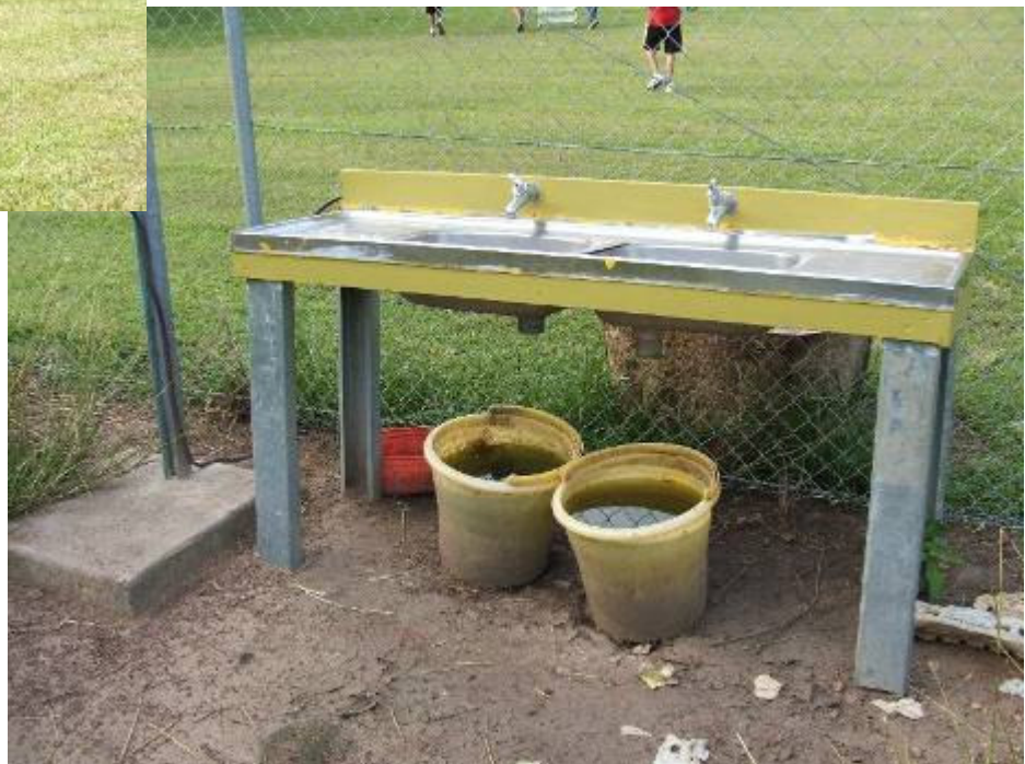
The new sink
